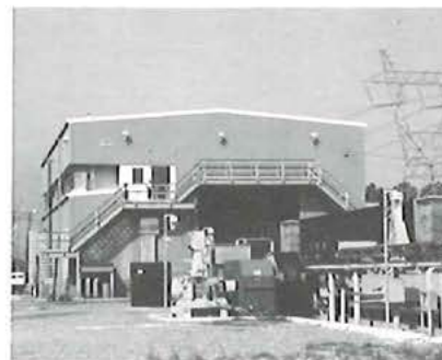
Aerated Storage Silo
