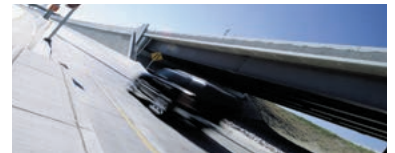
The American Road & Transportation Builders Association estimates coal fly ash use in roads and bridges saves $5.2 billion per year in U.S. construction costs.
